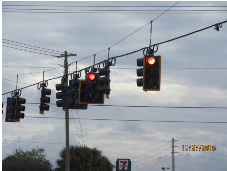
Figure 31 – Example of Yellow Reflective Sheeting at the Minton Road/Malabar Road Intersection
