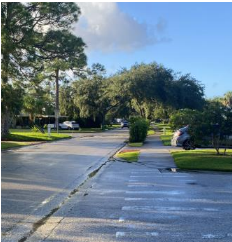
Pedestrian Ramp at Cambridge Drive & Tate Street
