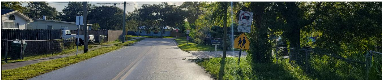
Existing Sidewalk Gap on Tate Street
