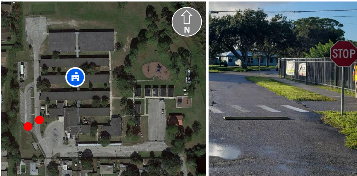
Existing Stop Signage and Stop Bar Locations
