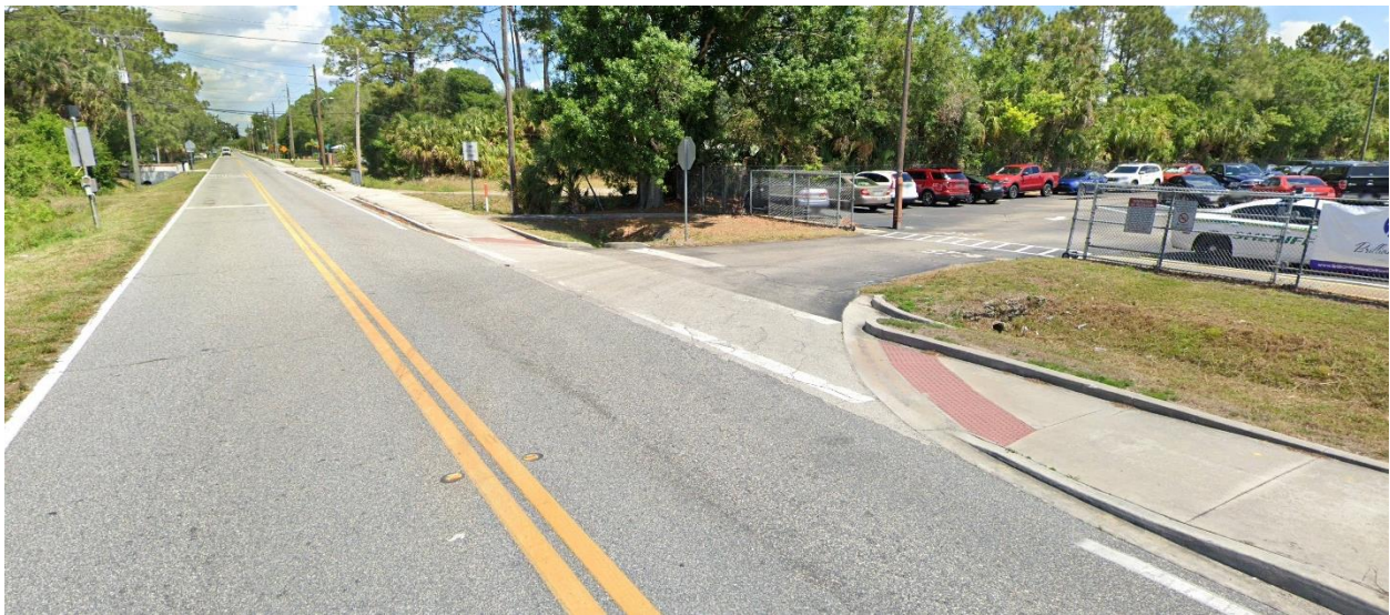
Existing Faded Crosswalk on Range Road at Southern School Driveway
