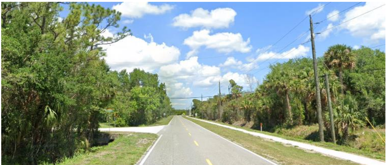
Existing Sidewalk Gap on Range Road
