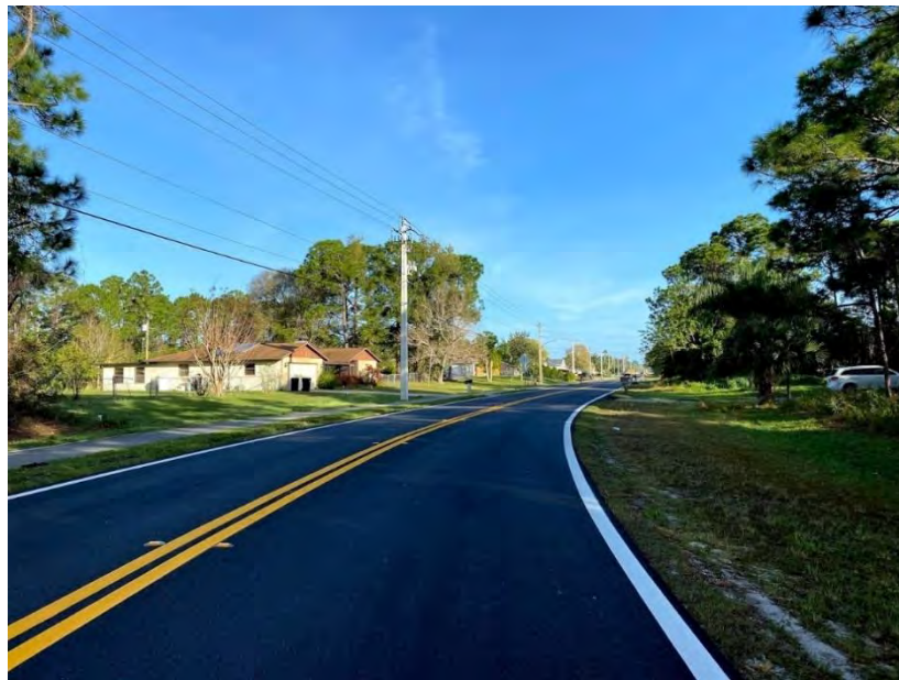
Eldron Boulevard North of Hatcher Street Facing North
