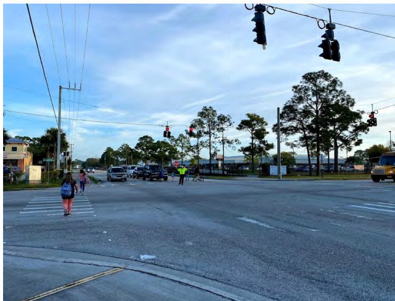
Faded Crosswalks at the Intersection of Jupiter Boulevard and Eldron Boulevard
