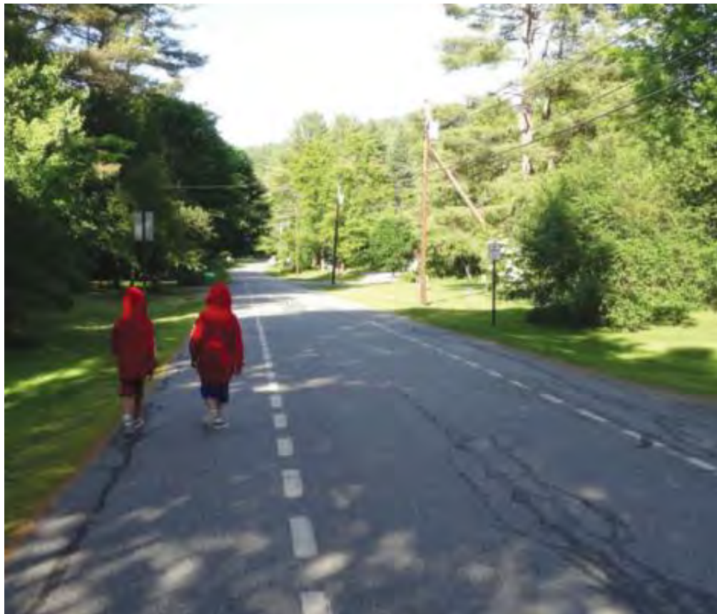
Advisory Shoulder Example from FHWA Small Town and Rural Multimodal Networks Report
