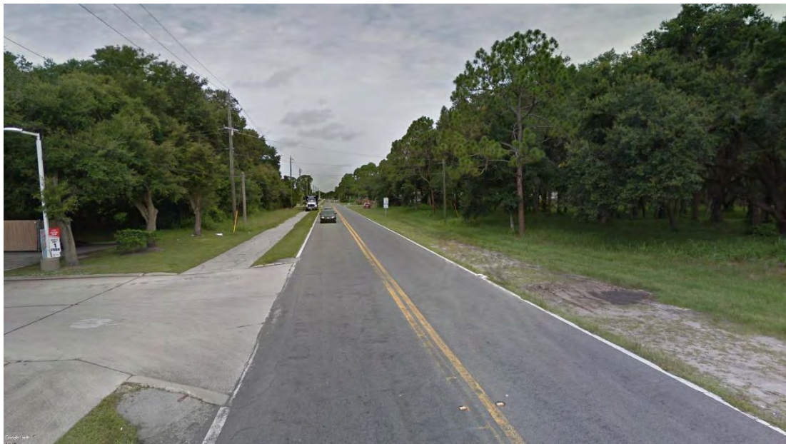
Americana Boulevard at Emerson Drive Facing North
