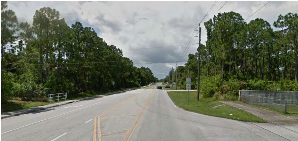
Sidewalk Gap Begins on Eldron Boulevard South of Jupiter Boulevard
