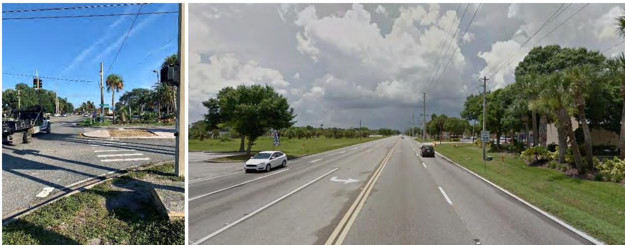
Sidewalks Gaps on Both Side of Wickham Road by Fountainhead Boulevard
