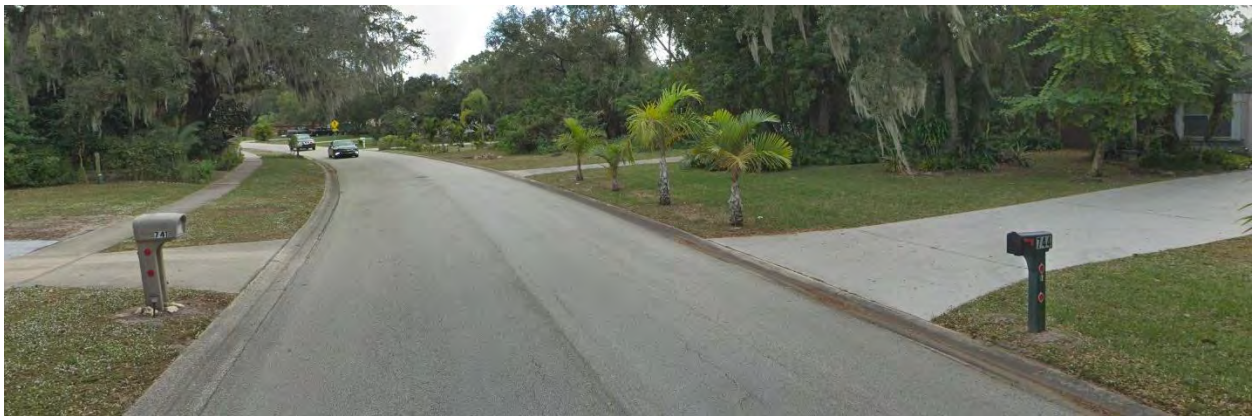
Sidewalk Gap Along Riviera Drive
