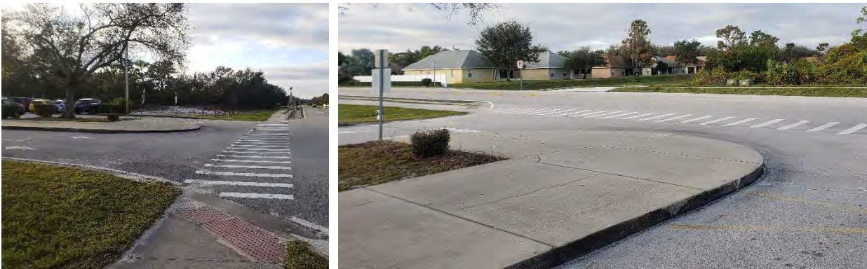
Existing Concrete Separator Between Bus Loop Driveway and Parent Drop-Off/Pick-Up Entrance Driveway
