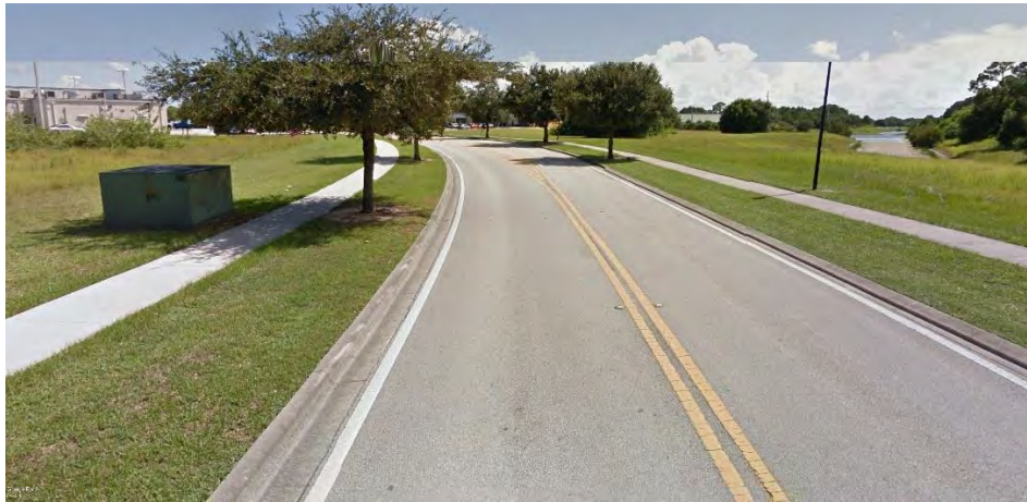
Existing Sidewalk Along Eldron Boulevard
