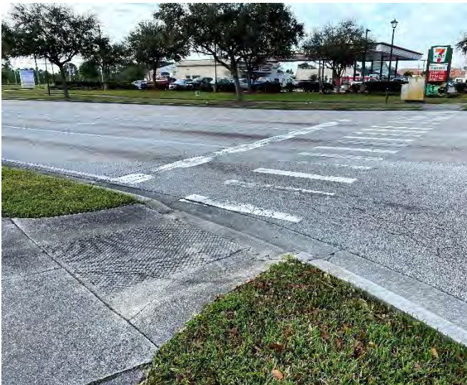
Restripe Crosswalks and Add ADA Compliant Pedestrian Ramps At the Intersection of Eldron Boulevard and Bayside Lakes Boulevard
