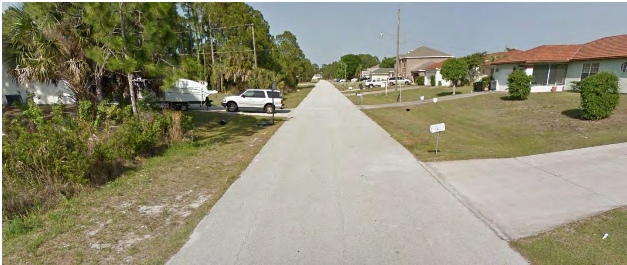
Sidewalk Gap Along Shrine Circle
