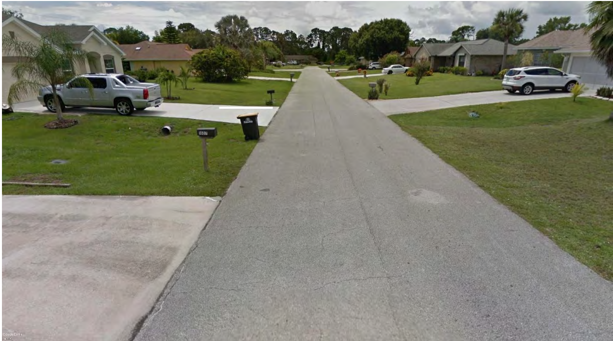
Lack of Sidewalk Along Elmhurst Circle
