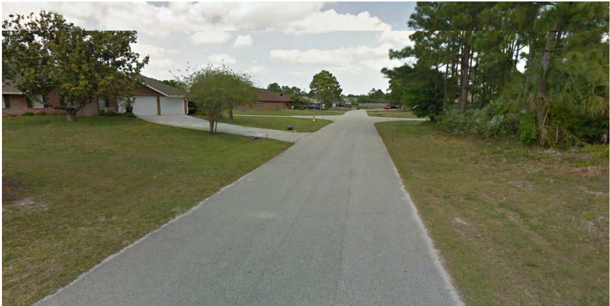
Sidewalk Gap Along Nemo Circle
