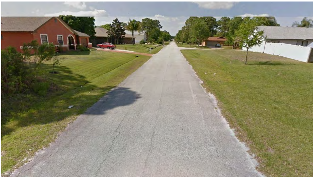
Sidewalk Gap Along Pelican Drive/Hyder Street
