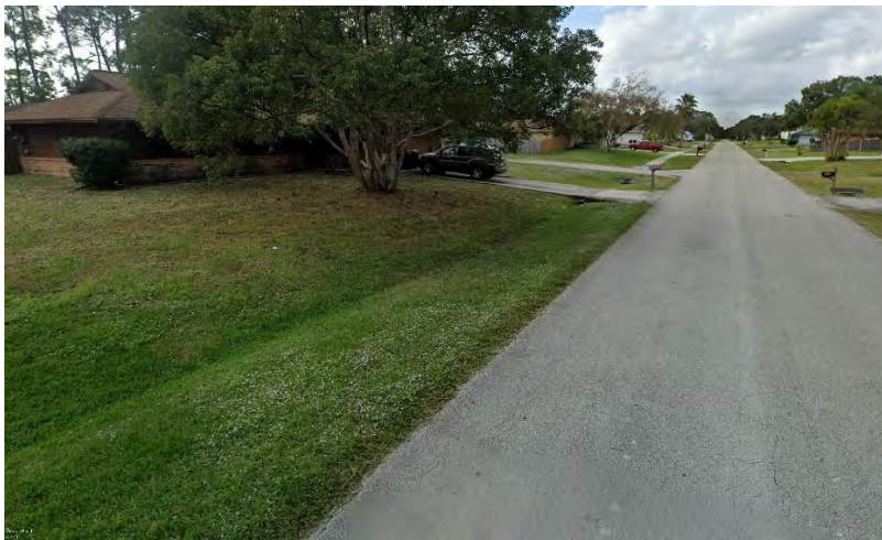
Sidewalk Gap Along Narragansett Street
