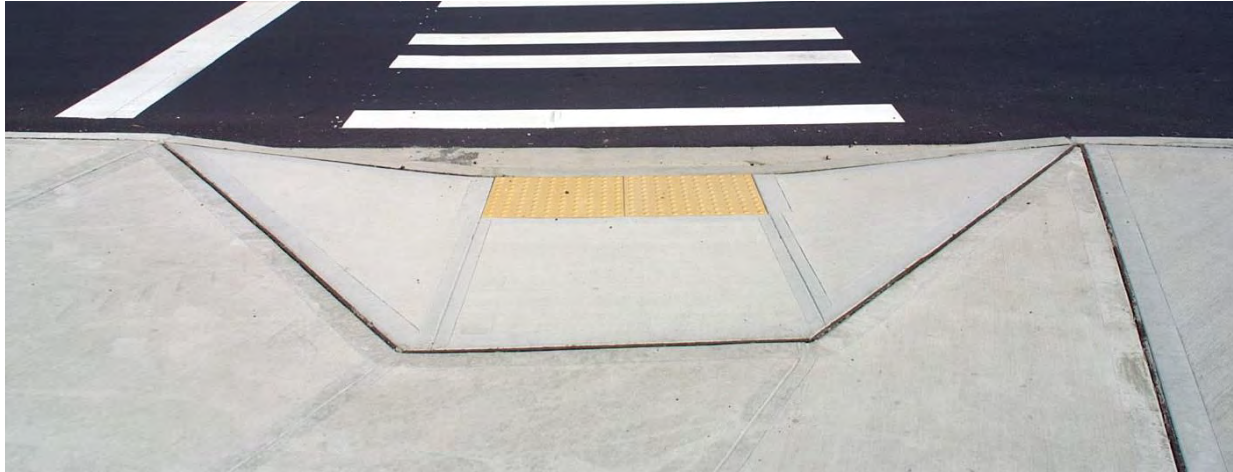
Perpendicular Pedestrian Ramp
