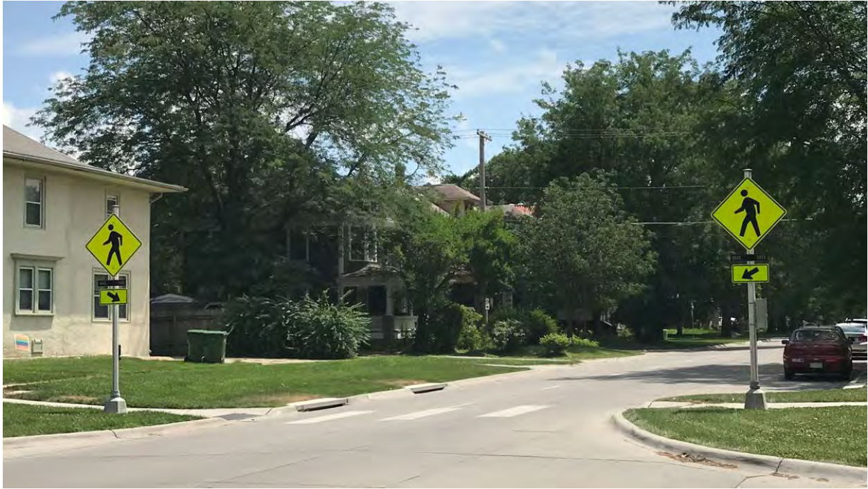
RRFB at an Intersection
