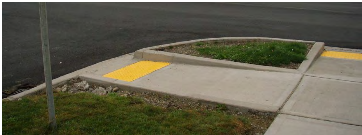
Unflared Perpendicular Curb Ramps
