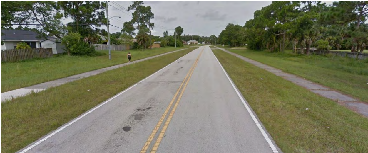
Existing Sidewalk Along Emerson Drive
