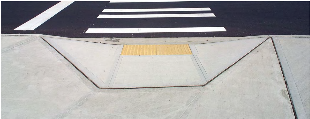
Perpendicular Pedestrian Ramp
