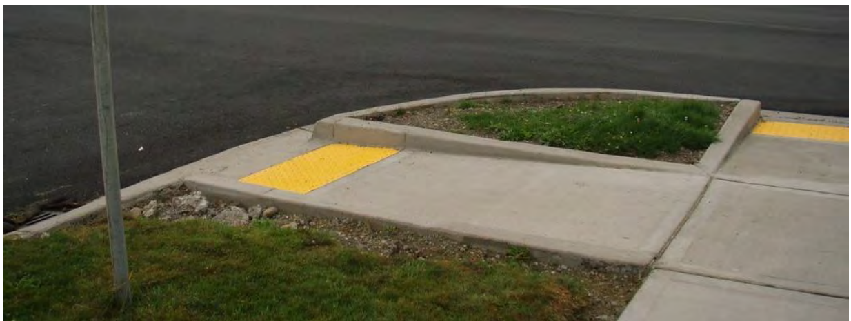
Unflared Perpendicular Curb Ramps
