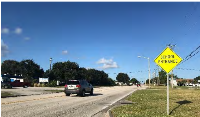
Existing 4-Lane Undivided Sarno Road
