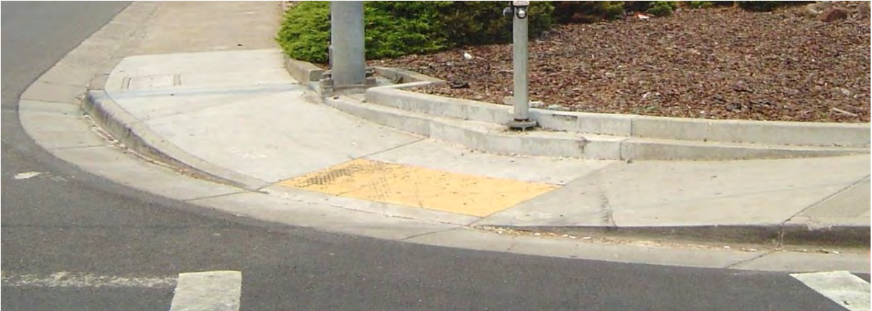
Diagonal Pedestrian Ramp
