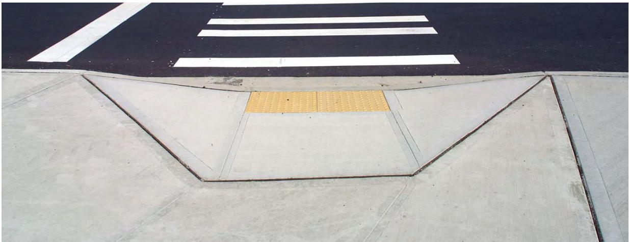
Perpendicular Pedestrian Ramp
