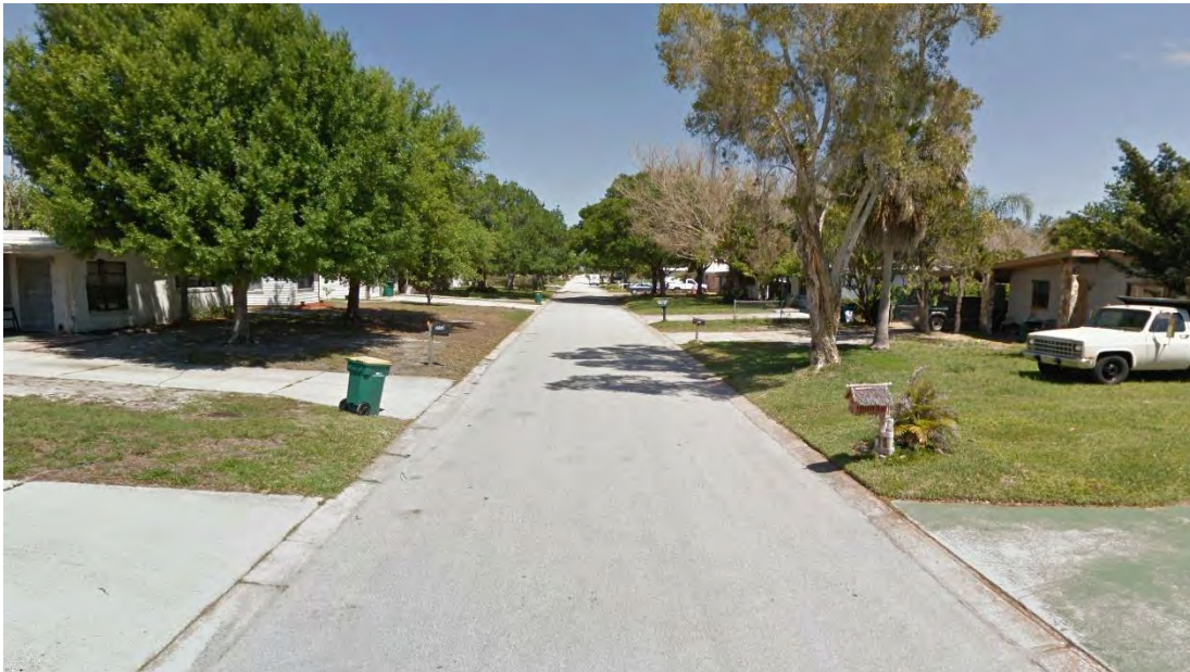
Cedarwood Drive Facing North
