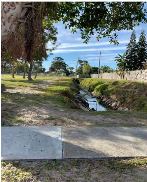
Canal in the School Study Area
