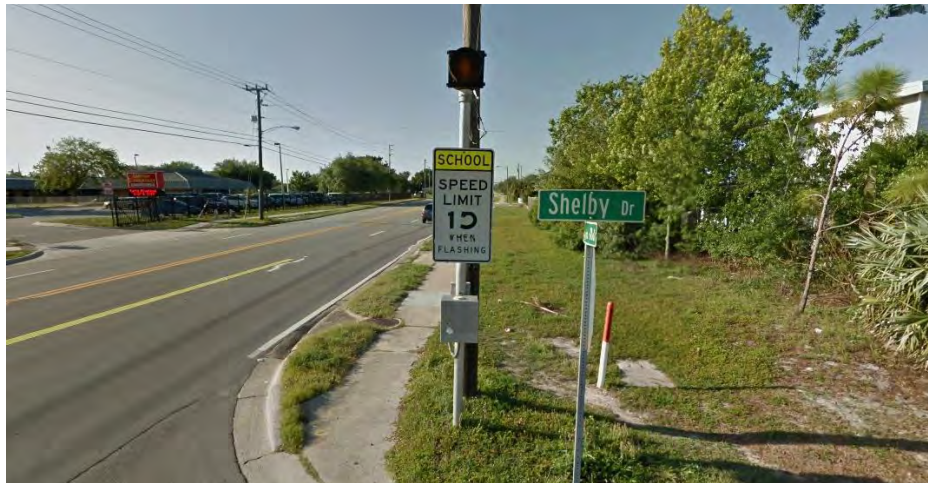
Existing School Zone Sign along Croton Road
