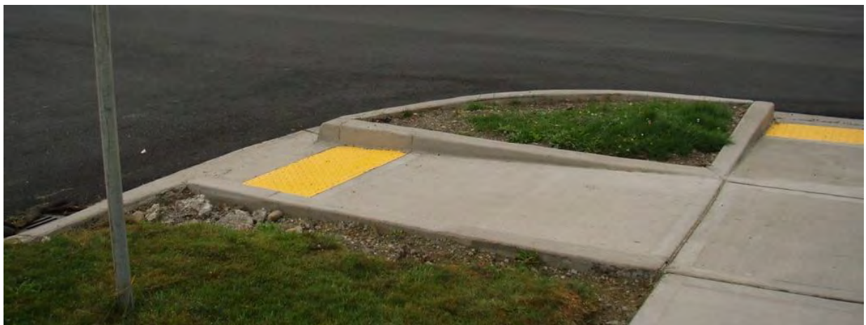
Unflared Perpendicular Curb Ramps
