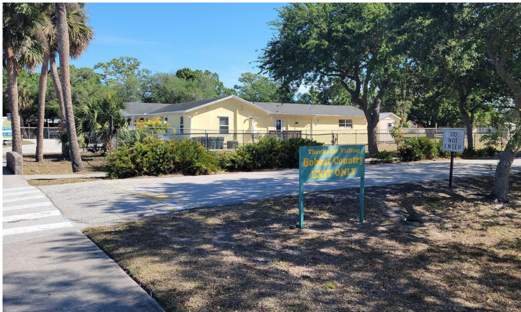
Existing “Do Not Enter” Signage at the Northernmost Driveway
