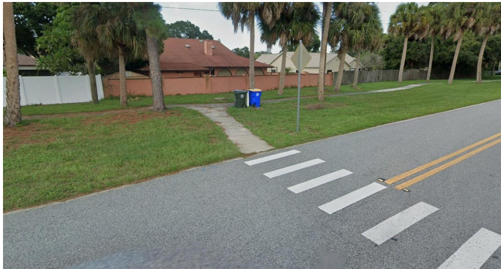
Existing Ramps on Barton Boulevard and St. Andrews Drive
