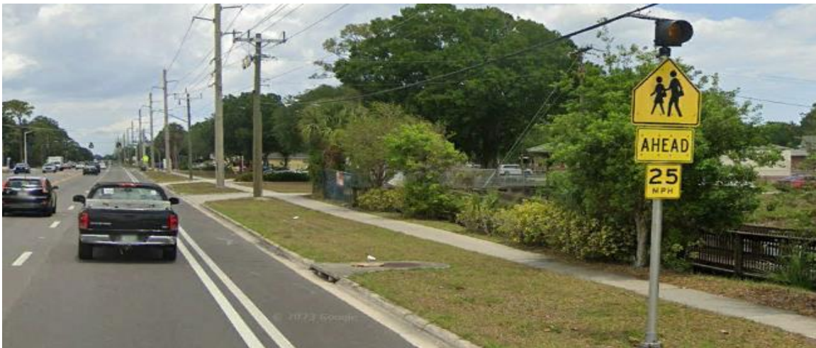
Existing Pedestrian Warning Signs along SR 519 (Fiske Boulevard)
