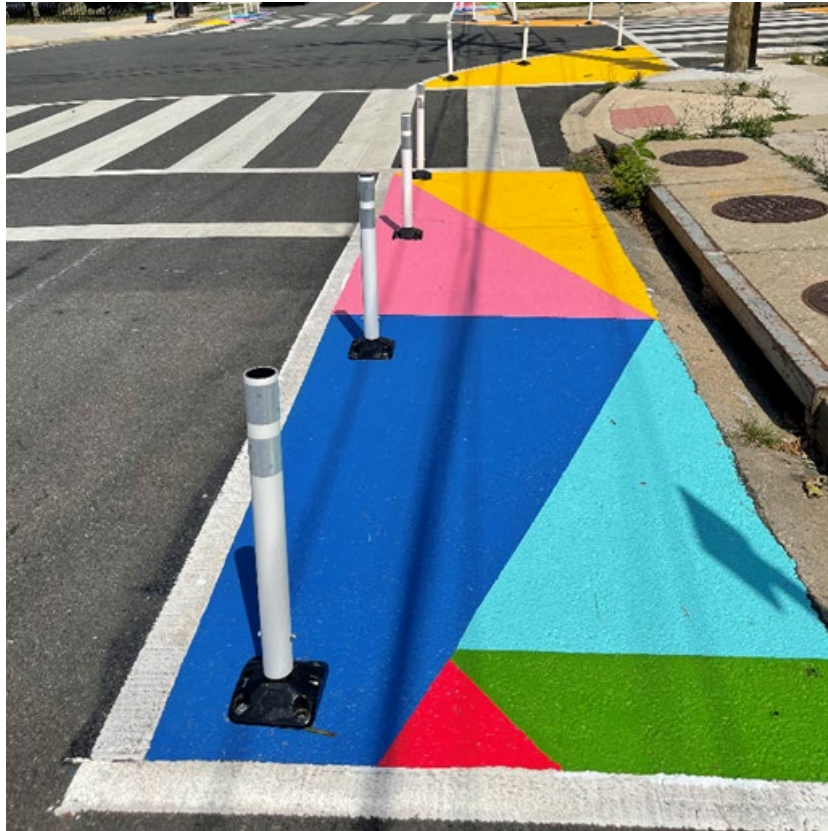
Curb Extension/Daylighting DDOT
