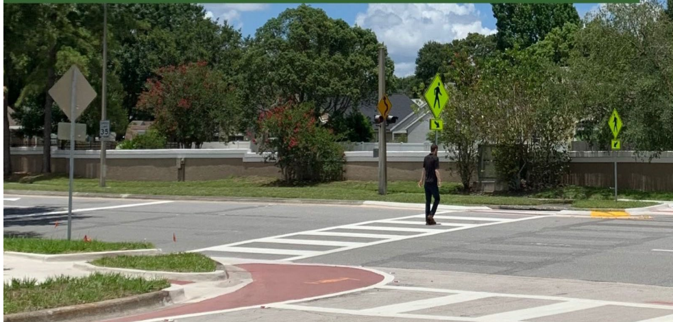
Painted Bulb Outs & Side Street Crosswalks
