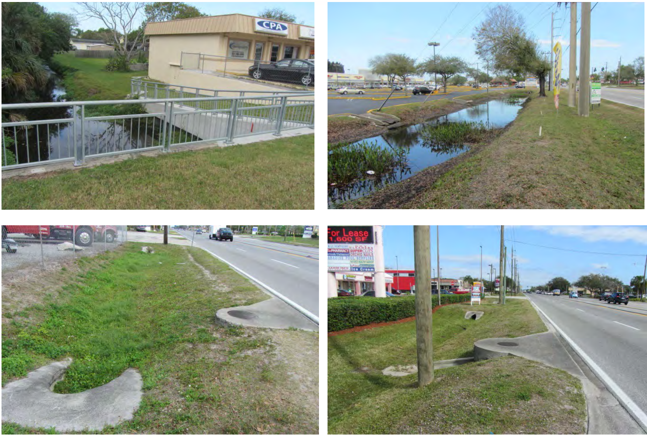
Figure 5: Existing Drainage Features along Wickham Road
