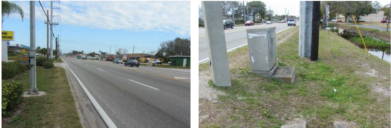
Figure 4: Adjacent Utilities along Wickham Road
