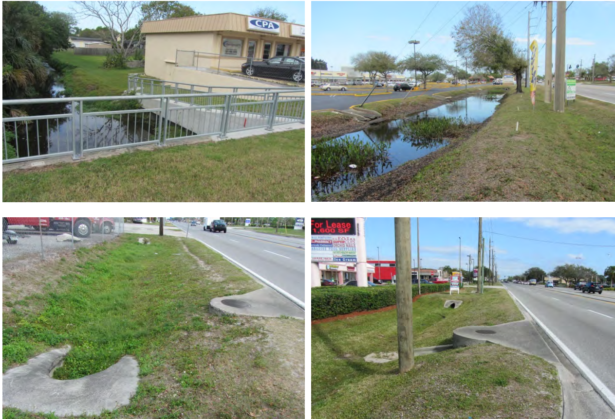
Figure 3: Existing Drainage Features along Wickham Road
