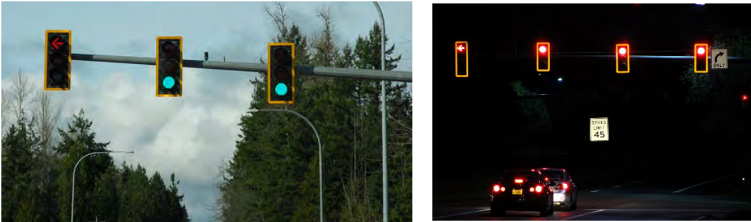
Figure 30: Retroreflective Signal Head Backplates
