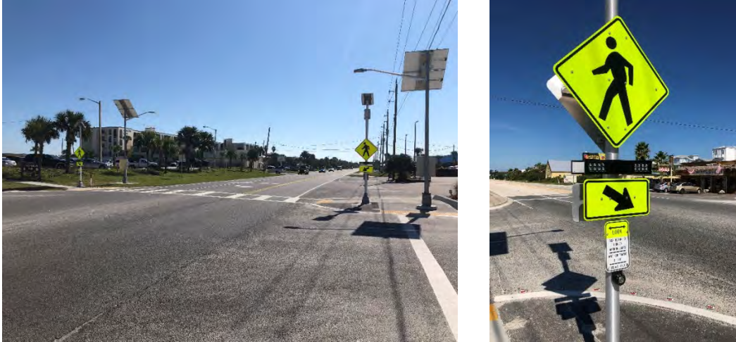
Figure 28: Retroreflective Rectangular Flashing Beacons
