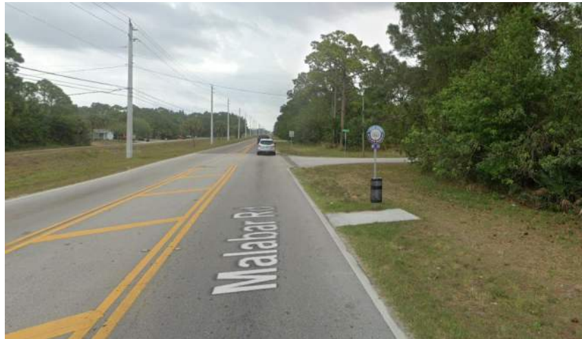
Figure 6-5: Western Side of Malabar Road with Sidewalk Gaps
